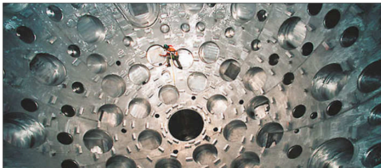
Construction worker inside National Ignition Facility target chamber.
